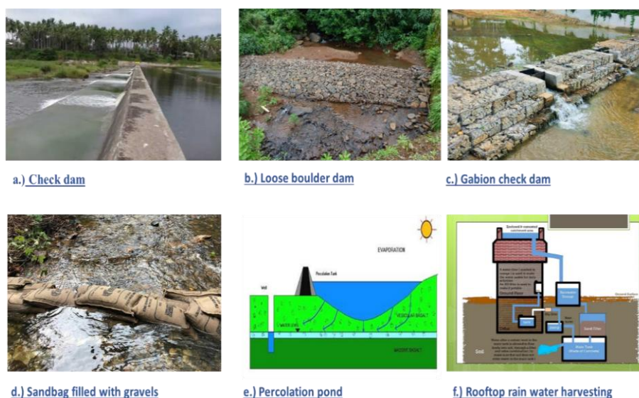
Fig. 4. Structures used for water harvesting
