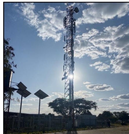
Fig. 14. Telecommunication towers built near municipal facilities
