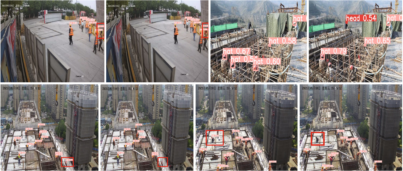
FIGURE 9: Detection pictures. Use for different work environments. Good at detecting small and dense targets.
